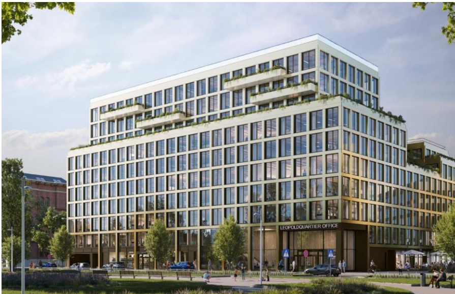
PORR is general contractor of the LeopoldQuartier OFFICE in Vienna © squarebytes
