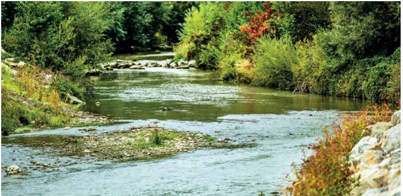
The Fahrafeld flood retention basin provides greater flood protection for communities in the Triesting Valley.
